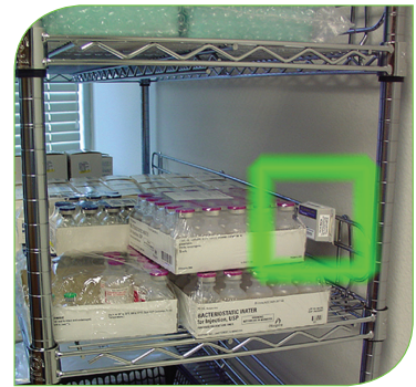
FlashLink wireless sensor monitors temperature in QuadraCare's clean room
